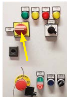
With electric indicator and particle counter Fig.19
