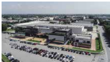
MP Filtri Headquarters in Milan
